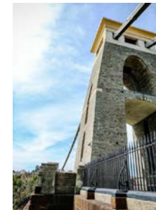
8. Clifton Suspension Bridge, Bristol
